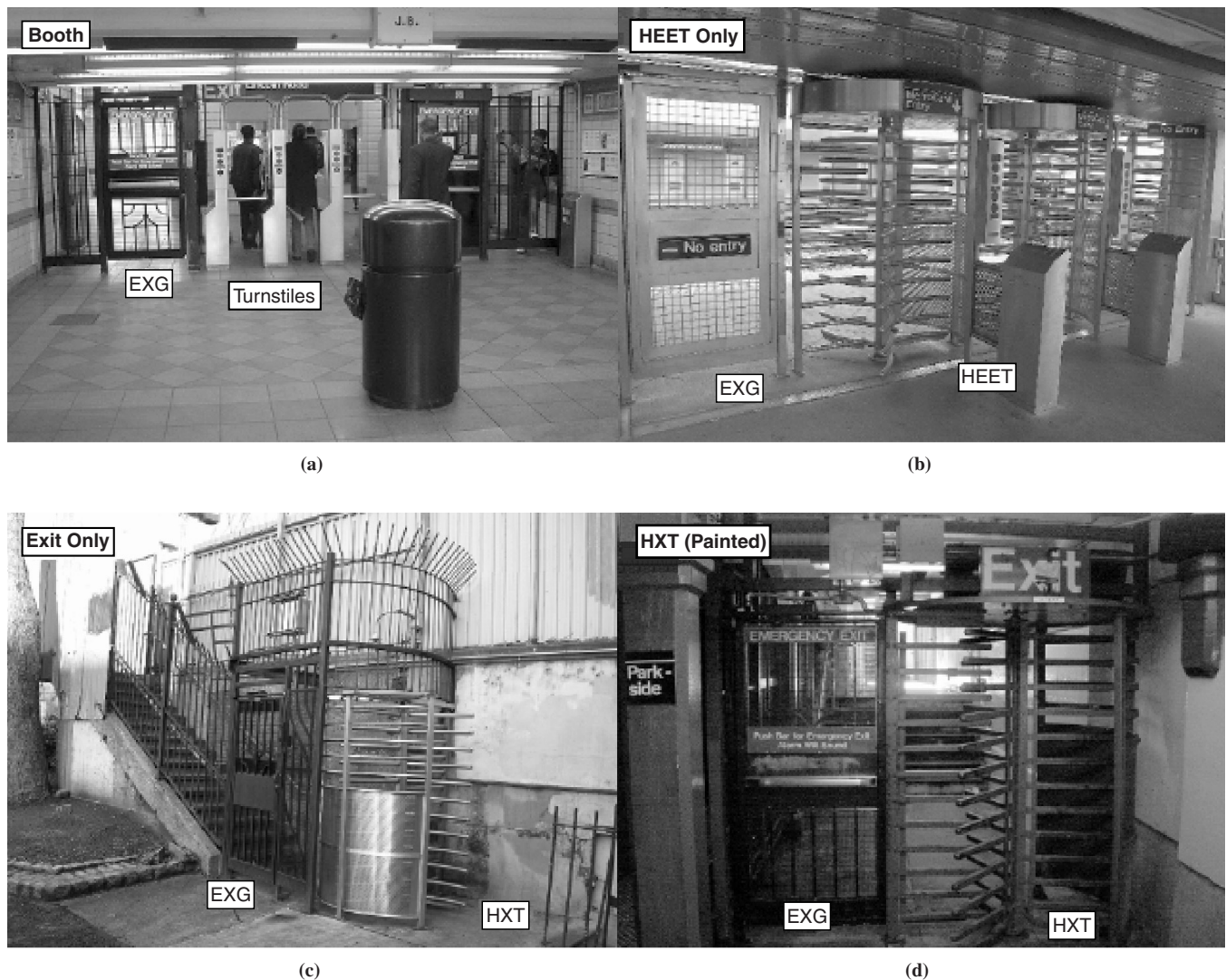
FIGURE 1 NYCT fare control areas featuring (a) three low turnstiles and two EXGs at Cortelyou Road Station on the Brighton Line (paid side), (b) two HEETs and one EXG in an unstaffed area at Howard Beach–John F. Kennedy Airport on Rockaway Line (unpaid side), (c) exit-only (unpaid side) with one high exit turnstile (HXT) and one EXG, and (d) exit-only (paid side) with an older-style painted HXT and one EXG.
